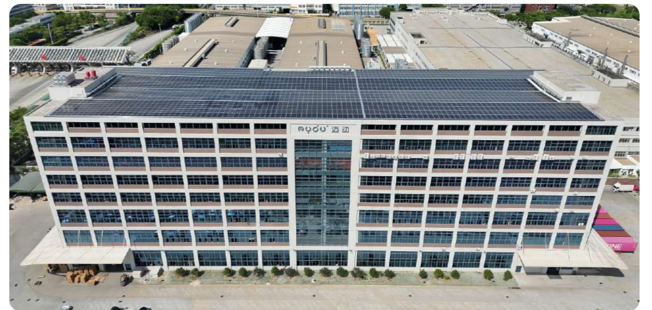
Project Name : Maidun Co.,Ltd.(Xiamen) BIPV rooftop solar power project Installed Capacity : 5.0MW
