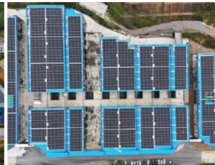
Project Name : Yunfu Stone City, Yunfu Guangdong Installed Capacity : 5.99MW
