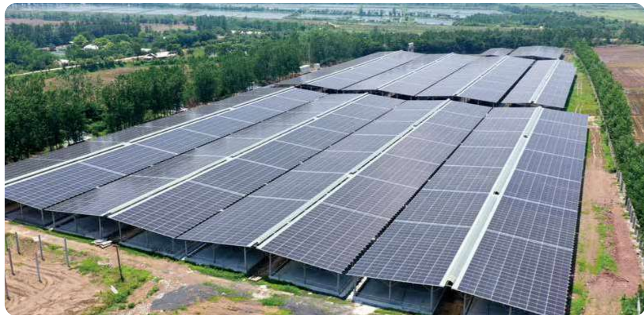
Project Name : Lingnan Beef Cattle Industrial Cluster, Anqing, Anhui Installed Capacity : 24MW
