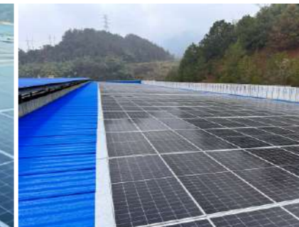
Project Name : Fujian Cable Manufacturing Factory Rooftop Solar PV BIPV Project Installed Capacity : 450KW
